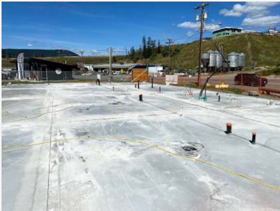
Beginnings of the cannabis facility
