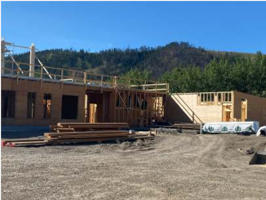
Administration Building under construction
