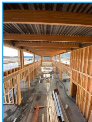
The interior of the new WLFN administration building.
