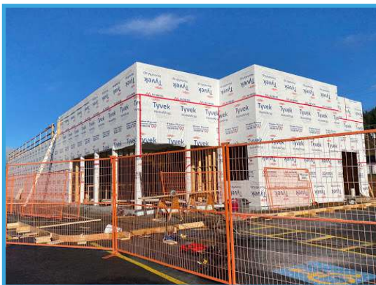
The new Sugar Cane Cannabis Facility, currently under construction.
