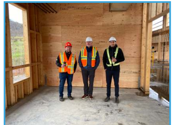
WLFN Chief Administration Officer Aaron Mannella, Grant, and Chief Willie Sellers in the new Administration Building.
